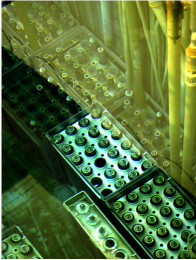
Fig. 1 Spent fuel in MARIA reactor storage pool.
